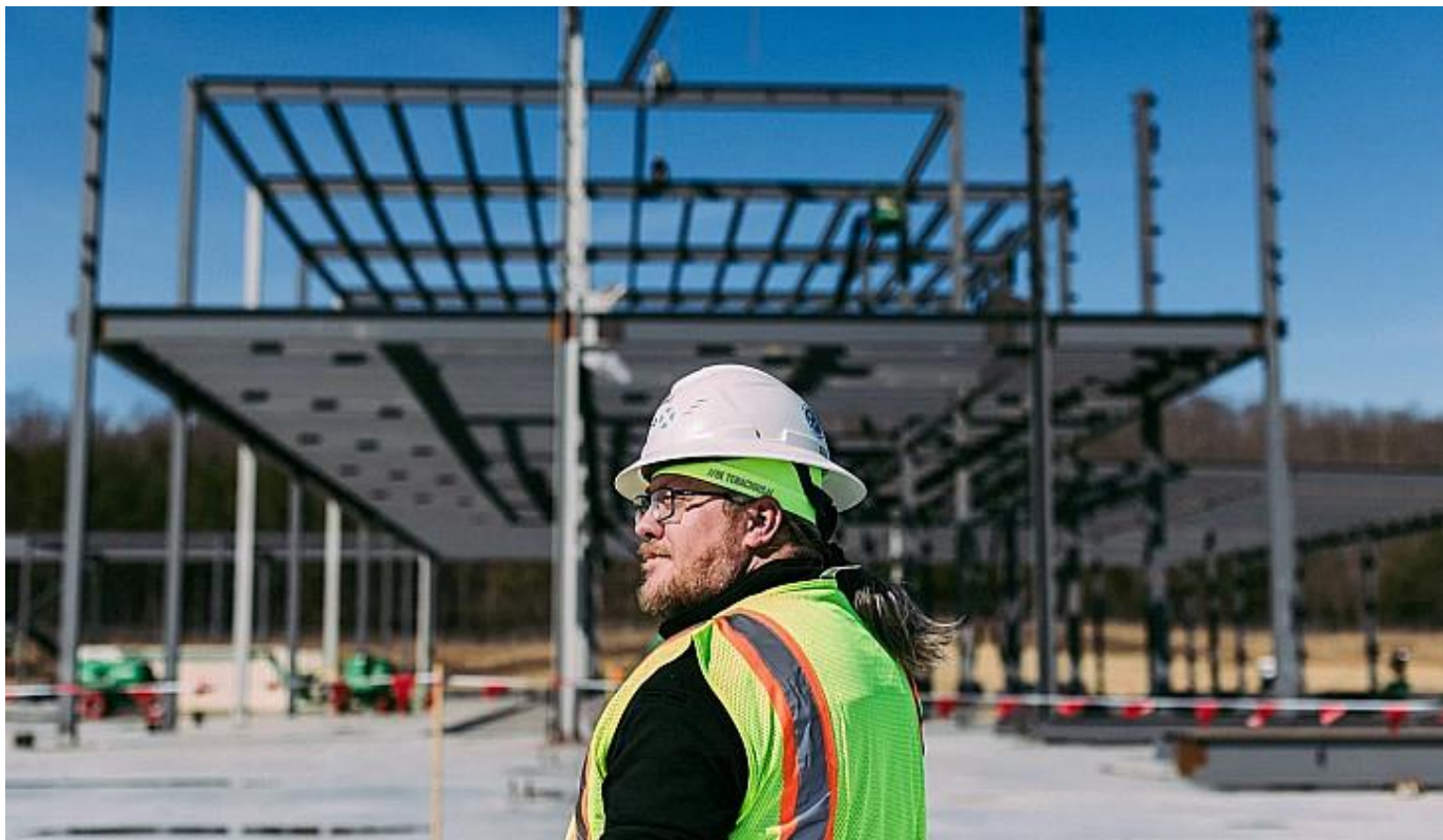
Image: The facility is under construction in Tennessee (X-energy)
